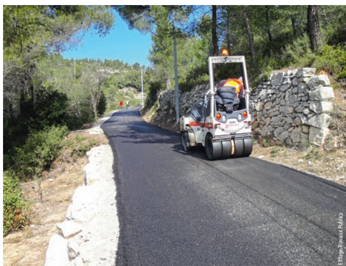
Photo 5 Compactage de l'enrobé Biocold Compacting of Biocold asphalt
