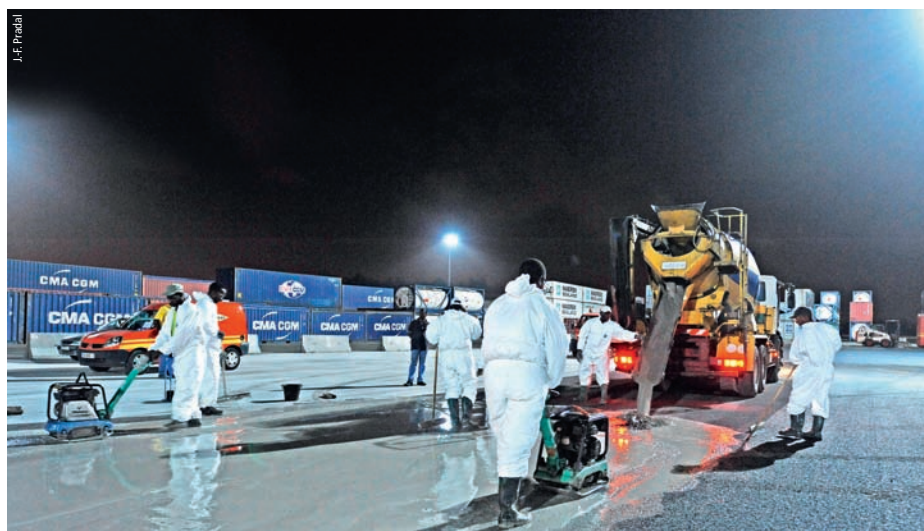
Photo 5 Chantier percolation Percolation (leaching) worksite
