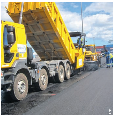
Photo 3 Application des enrobés Application of asphalt
