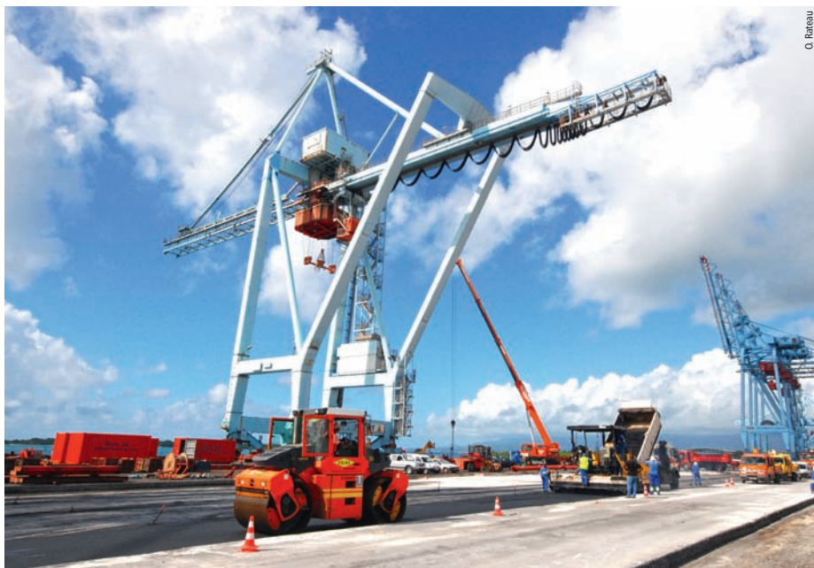
Photo 2 Application des enrobés Application of asphalt
