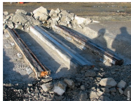
Photo 7 Poutre béton rail acier Concrete beam, steel rail
